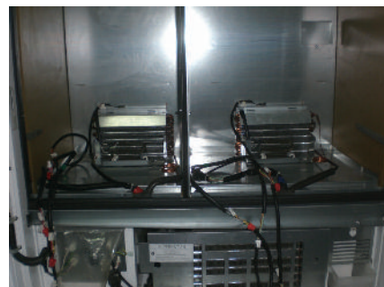
Fig 13b. Overall compartment condition after chute removed.
