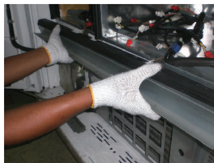
Fig 15b. Remove drain lower trim
