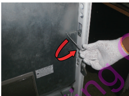
Fig 1. Open inner door To open inner door, lift and slide lever (inner door lock)
