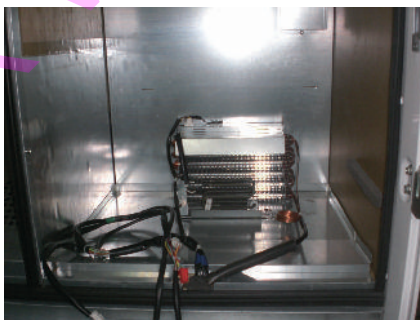
Fig 13a. Compartment condition after chute removed.
