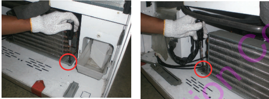
Fig 19a. Remove screws of refrigeration unit
