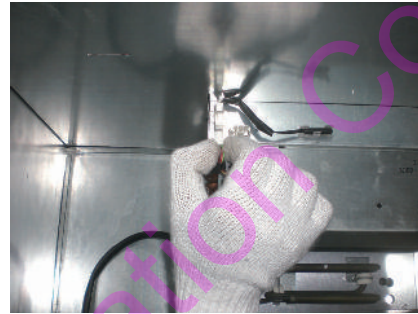
Fig 14b. Remove sensor temperature connector.
