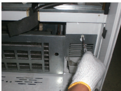
Fig 18a. Remove sponge and plate condenser guard
