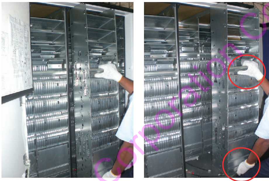
Fig 7a. Remove rack unit (lift and draw out rack unit from rack rail).
